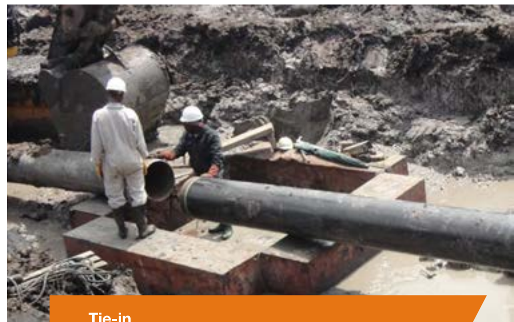
Excavating to 4 meters below ground level for tie-in
