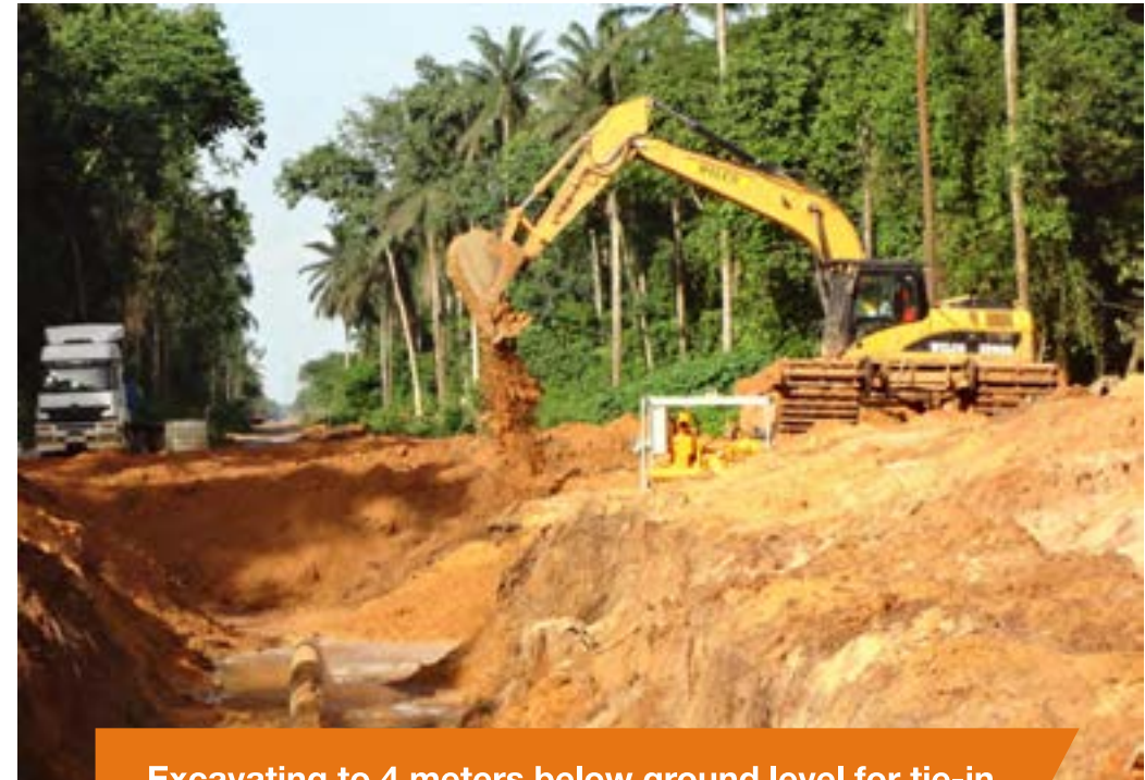
Excavating to 4 meters below ground level for tie-in
