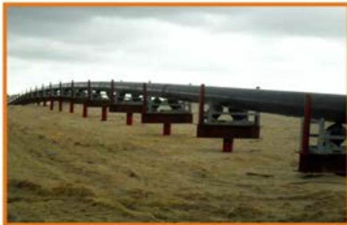
ESCROVOS RIVER CROSSING, PICTURE OF PRODUCT 24" PIPES IN OVERBEND ROLLERS POSITION PRIOR TO PULL BACK
