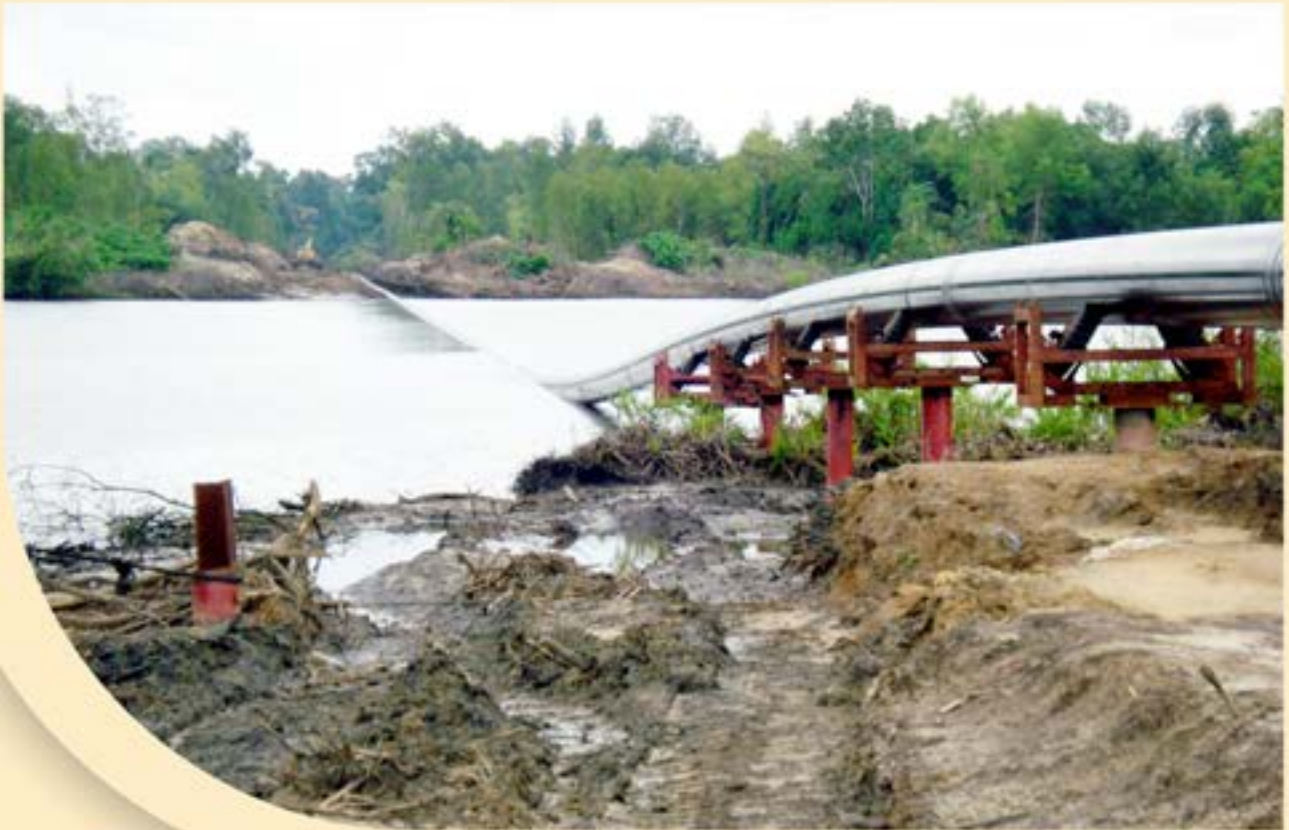
24INCH PIPE ON ROLLERS AT EXIT LOCATION FOR ERC PROJECT
