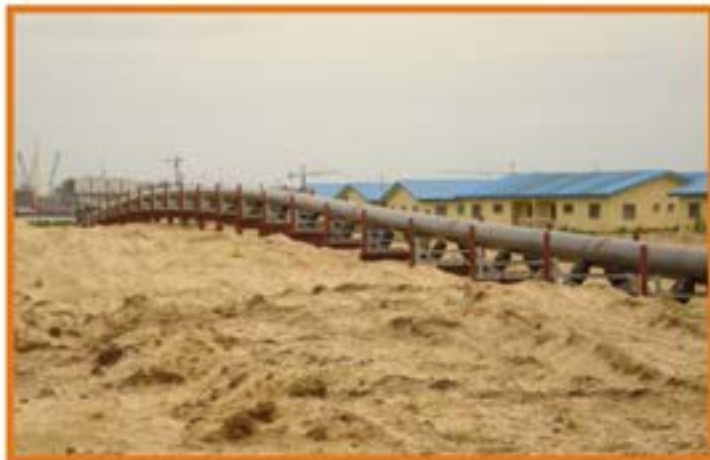
ESCROVOS RIVER CROSSING, PICTURE OF PRODUCT 24" PIPES IN OVERBEND POSITION PRIOR TO PULL BACK
