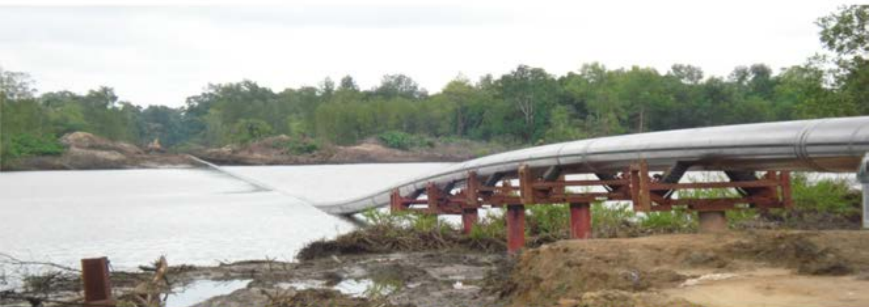
ERC HDD PROJECT , PICTURE SHOWING PIPE AFLOAT ON WATER PRIOR TO HDD PULL BACK.
